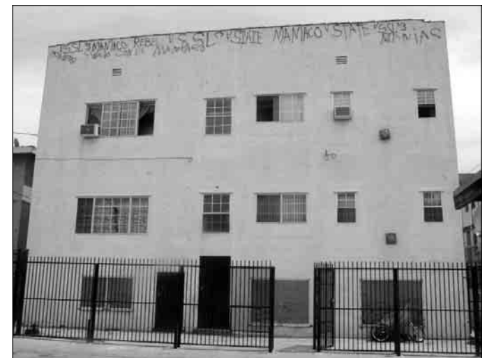
Graffiti marks the top of the back of the East Los Angeles apartment building once inhabited by the family of Michael Jackson's accuser.
